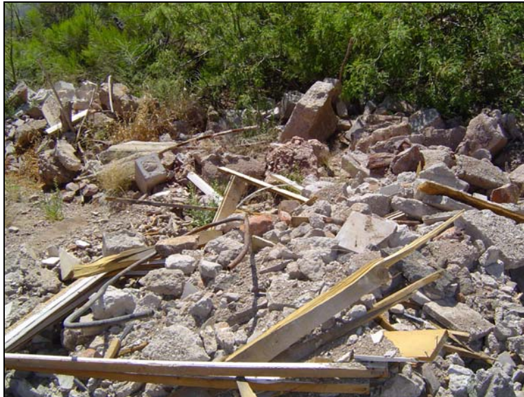
Drywall and concrete debris located near the northeast end of building north of parking lot.
