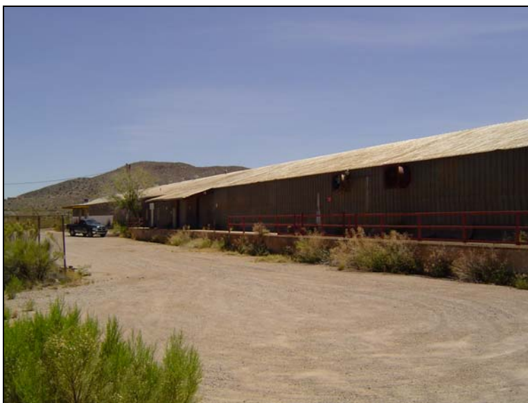
East side of building in parking lot – looking southeast.
