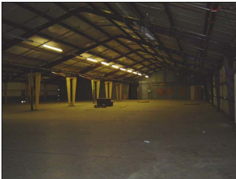
Inside south end of building looking north.
