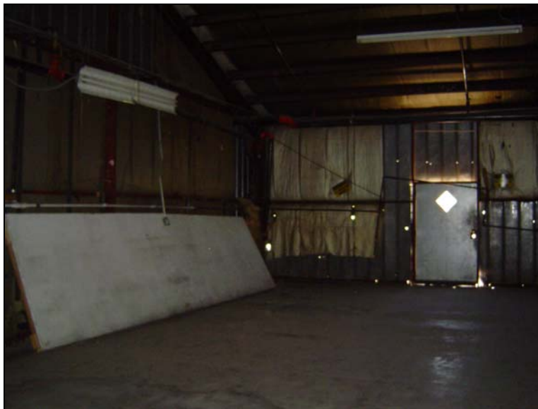
Inside middle of building.
