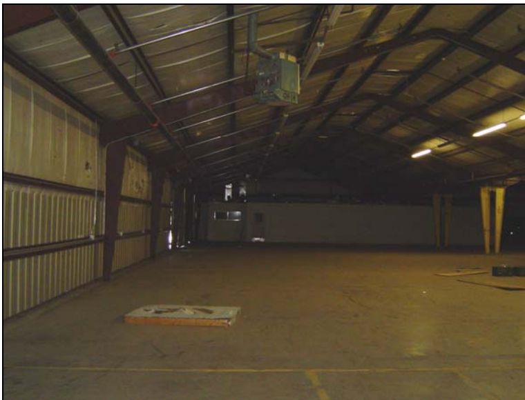
Inside south end of building looking south.
