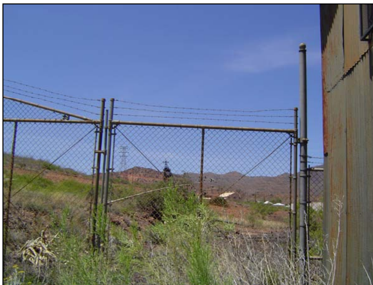
Outside along northwest side of building.
