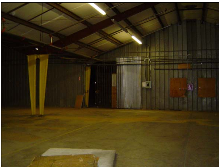
Inside south end of building looking west.
