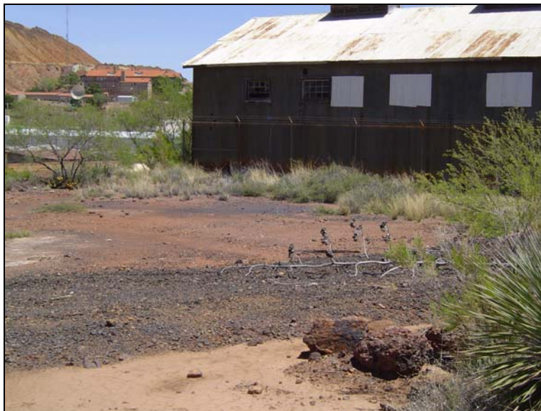
Stained soil and sparse vegetation located near northwest end of building.
