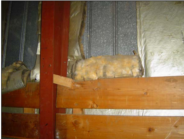
Insulation along west wall of building.
