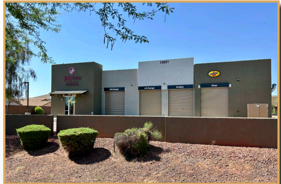
Construction As of June 2024
