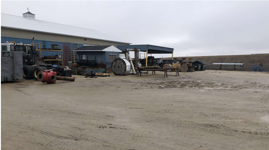
The yard has 2 steel overhangs with power
