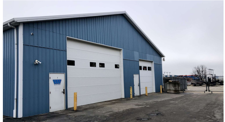
New overhead 18' x 12' overhead door can fit semi-trucks
