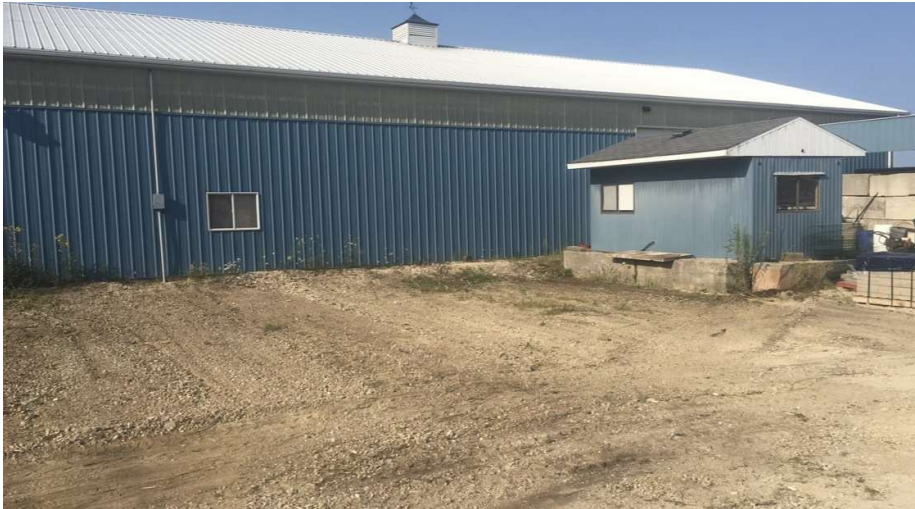
The back area has a foreman's office with AC, heat and electric
